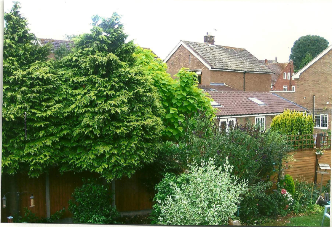
VIEW OF REAR EXTENSION AT 1 MONMOUTH ROAD, FROM, 102 GOSWELL END ROAD
